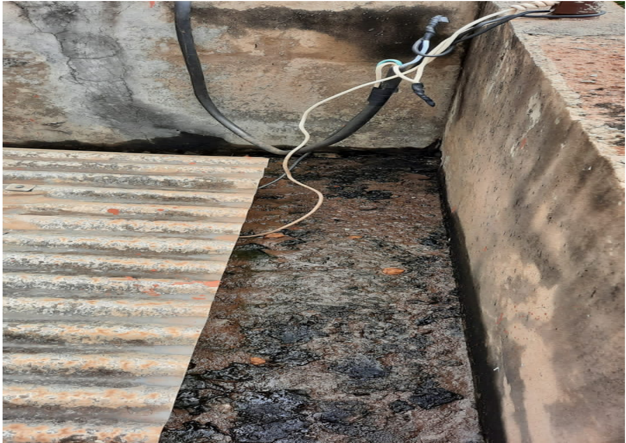
Pict. #3: Silt Deposit within Roof Drainage Channel (Algae Growth due to dampness in the drainage)
