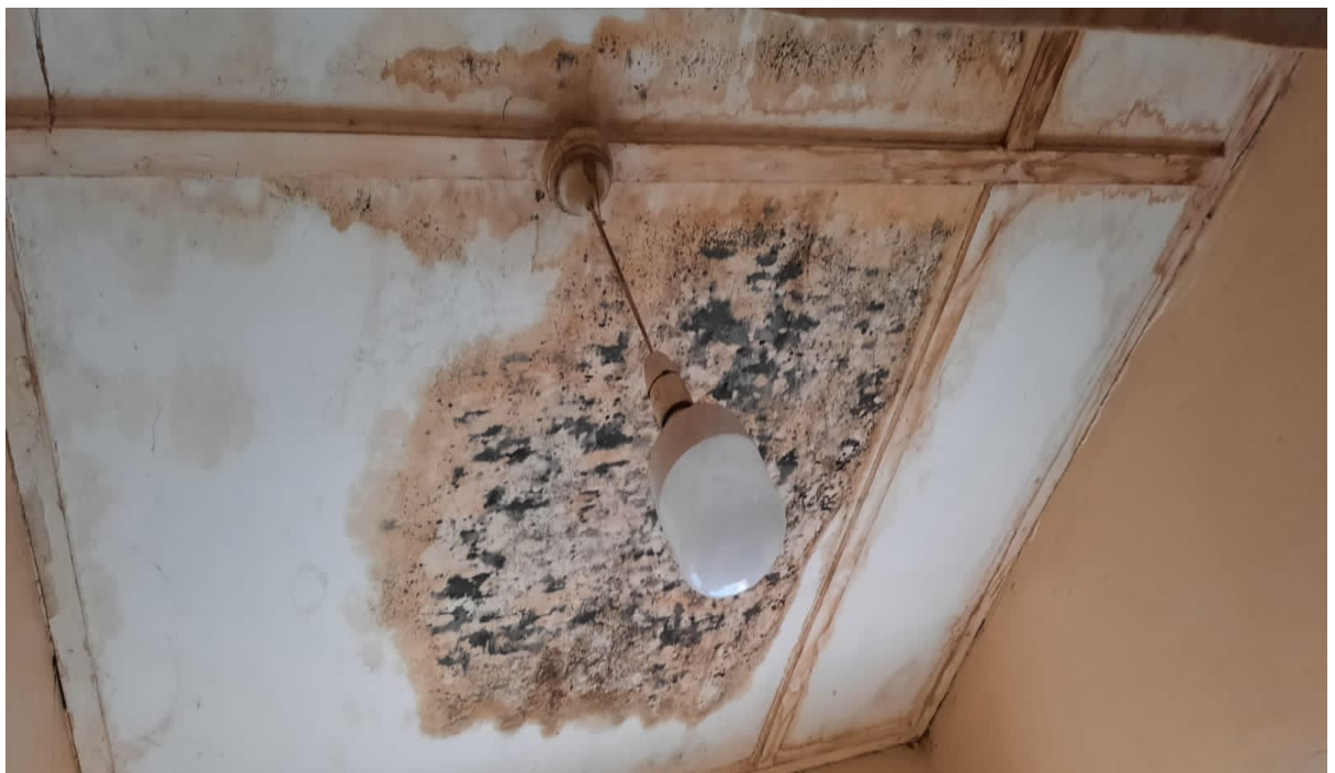
Pict. #4: Visible Deterioration in the Plywood Ceiling
